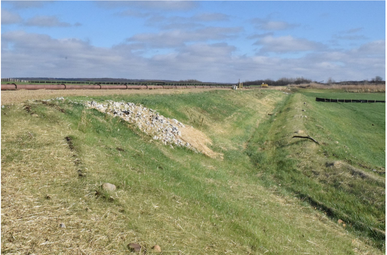
West downstream slope – filled area
