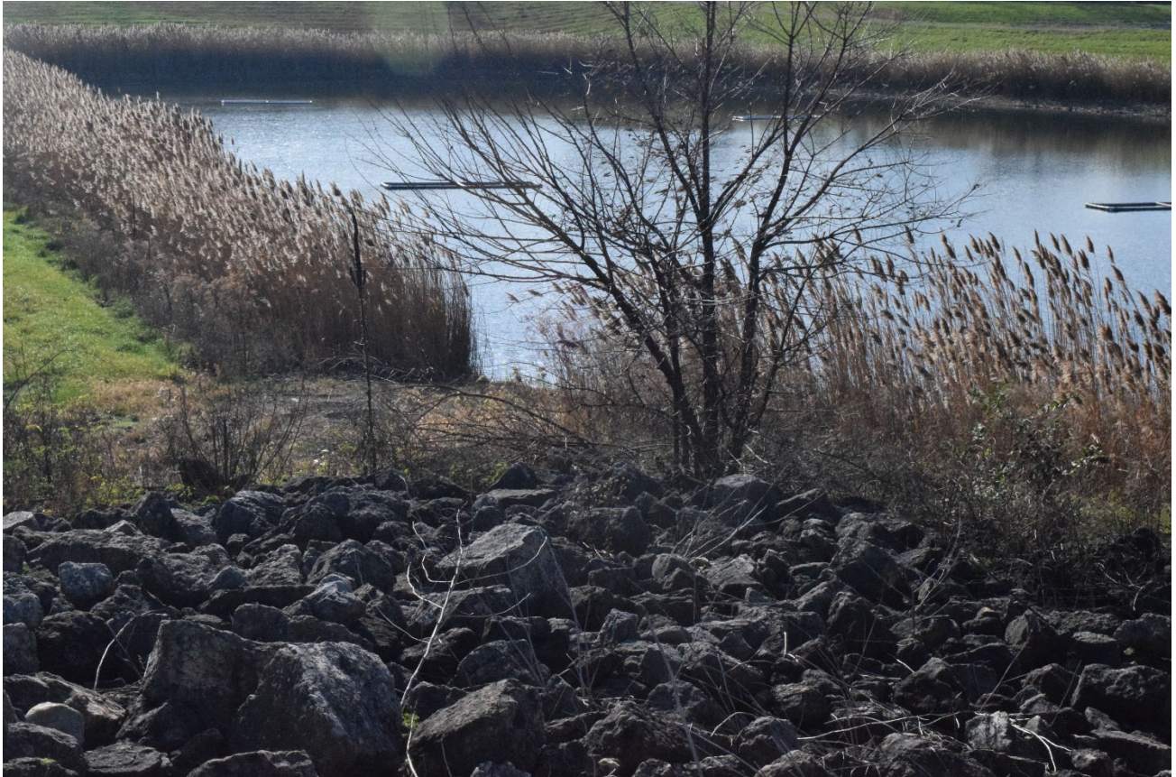
Secondary pond and outlet structure to river – spray/remove vegetation in riprap
