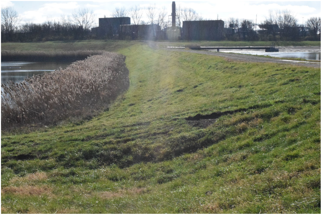
Primary pond – secondary pond separator berm
