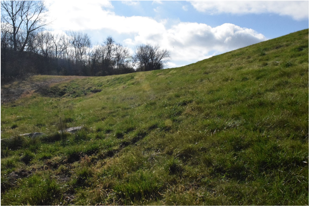
East exterior slope
