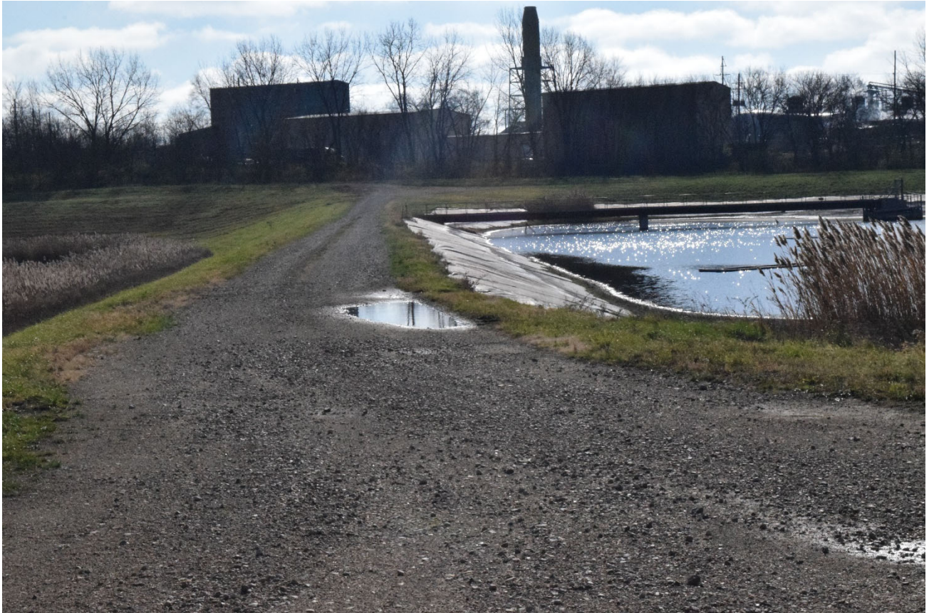
Primary pond – secondary pond separator berm
