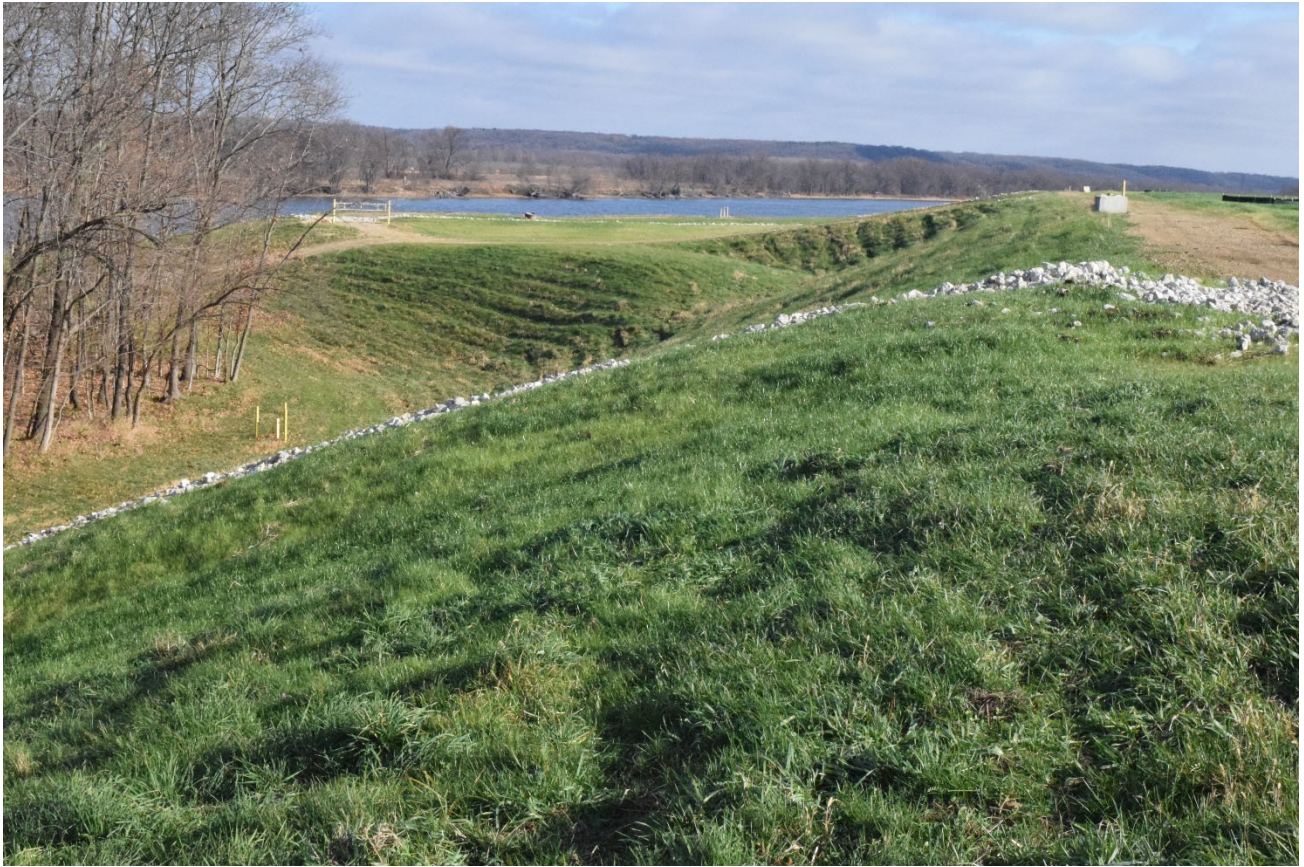
North side exterior
