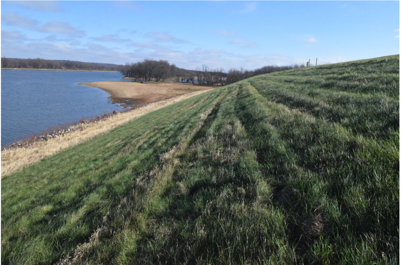
North side adjacent to river
